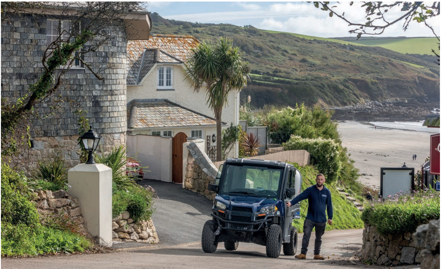
The Gatehouse was an important part of improving the approach to the hotel. It was built using granite and Delabole slate. The first floor contains a meeting/training room with a workshop underneath allowing the bin yard to be relocated to the recycling yard. Dan uses an electric buggy to transport the refuse to the top of the hill.
